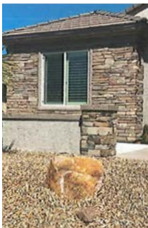
Front Courtyard Walls Section IV.B.9.C.
